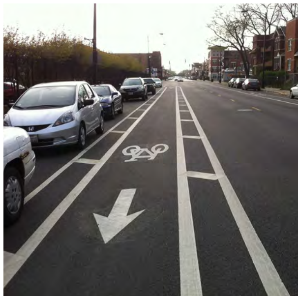
Figure 2.7 Buffered bike lane in Chicago. Source: Active Transportation Alliance.
